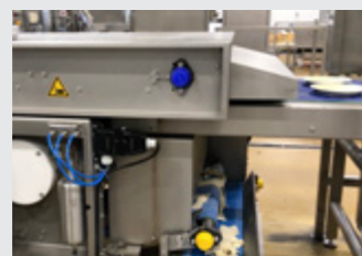
6 The outfeed system transfers quiches onto a conveyor belt. Rework dough is processed to a rework system.
